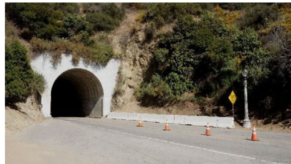
Mount Hollywood Tunnel
